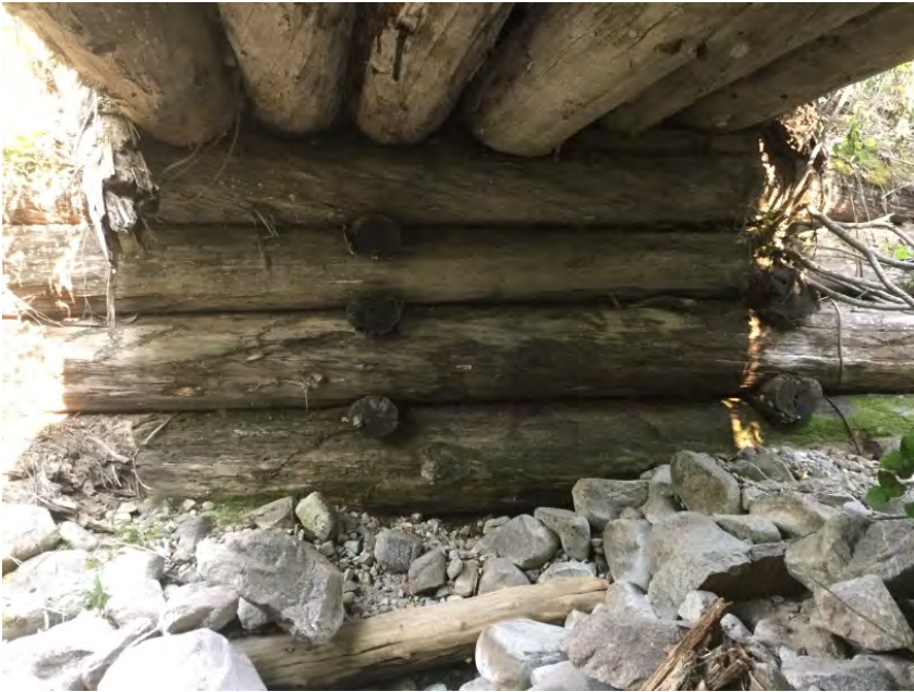
Right Bank Abutment when facing downstream
