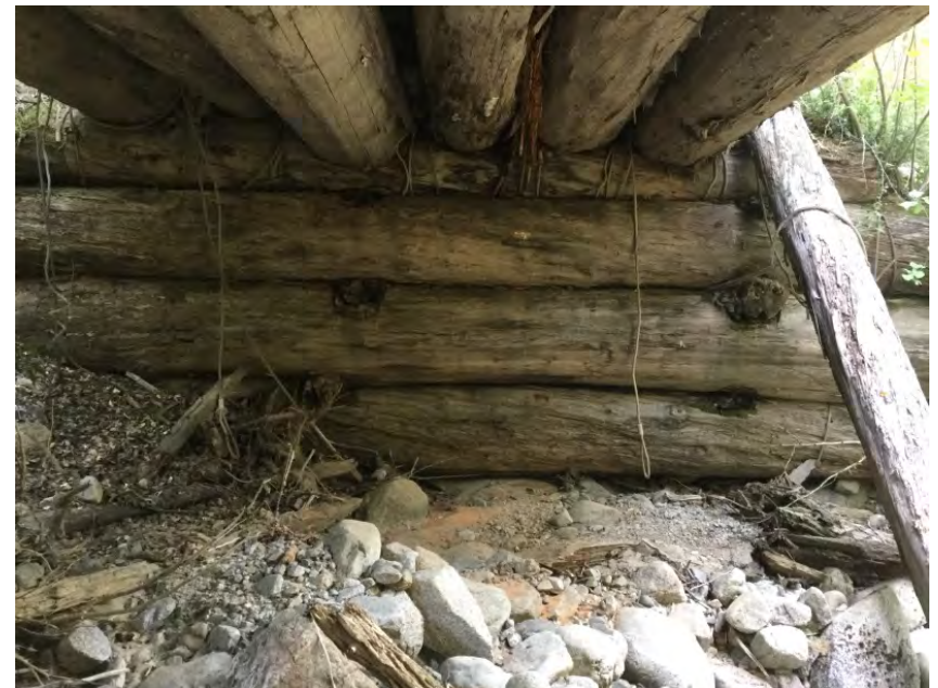
Left Bank Abutment when facing downstream
