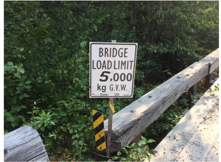
Load Rating Sign
